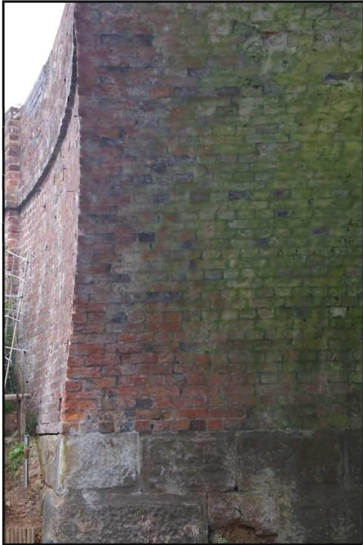
Fig 8: Bridge at Tardebigge; Worcester and Birmingham Canal
