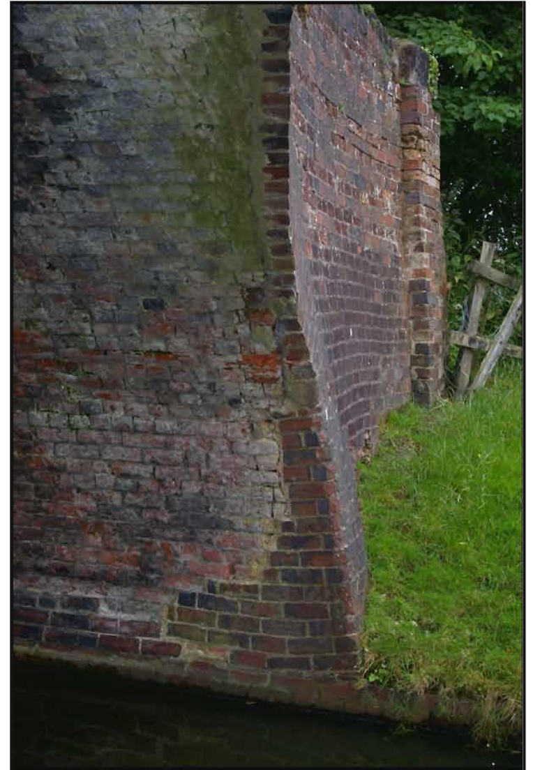
Fig 9: Bridge at Hockley Heath; North Stratford Canal
