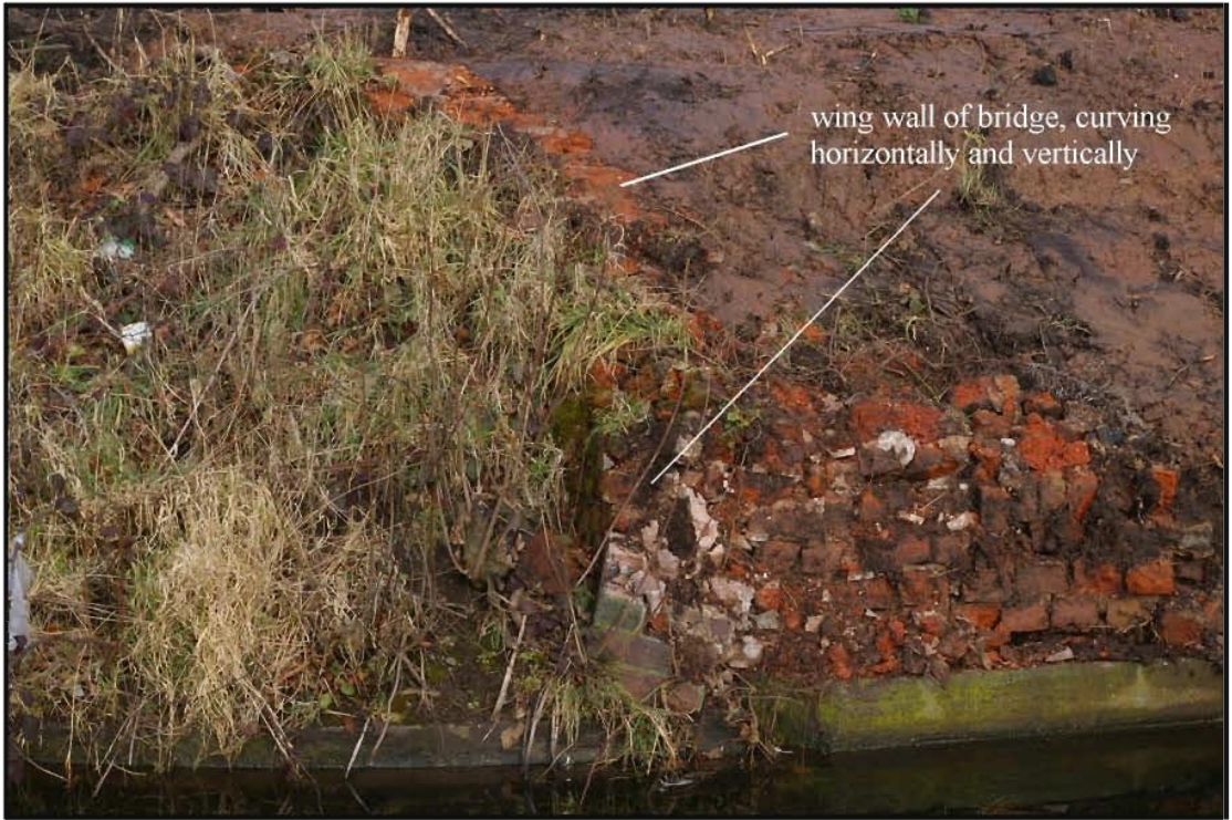
Fig 13: View of northern bridge abutment showing curving wing wall
