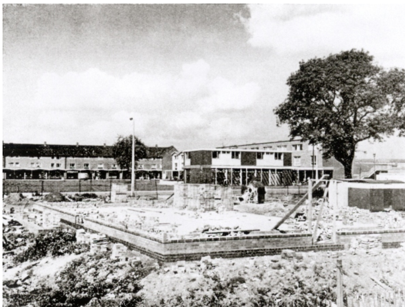
Starting work on St Alban's
